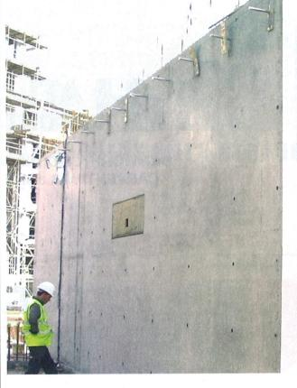
create unnecessary trip hazards for site workers, use additional formwork and leave the soffit face marked.
