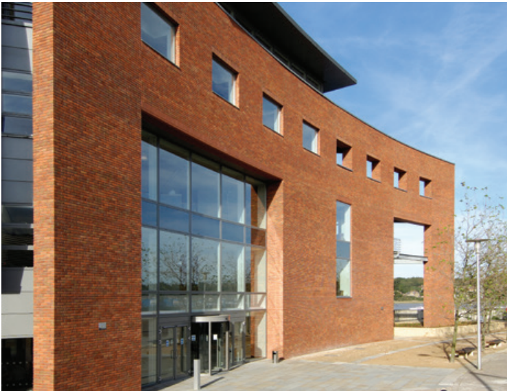
Special MDA Brackets Supporting Brickwork Curved on Plan
