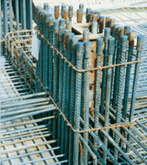
Column Construction using Tapered Thread Couplers
