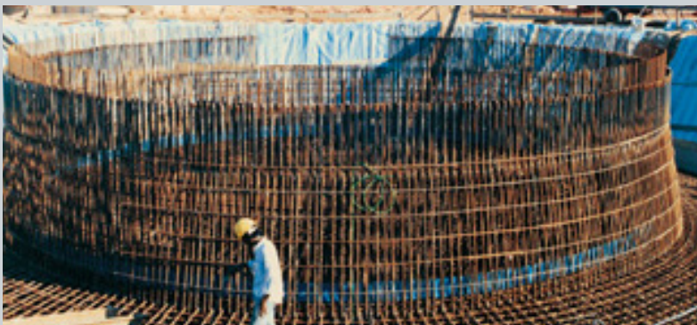
Tapered Thread Couplers used where density of rebar creates restricted access
