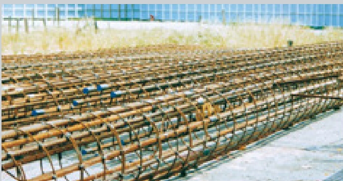
Pile Cage Connections
