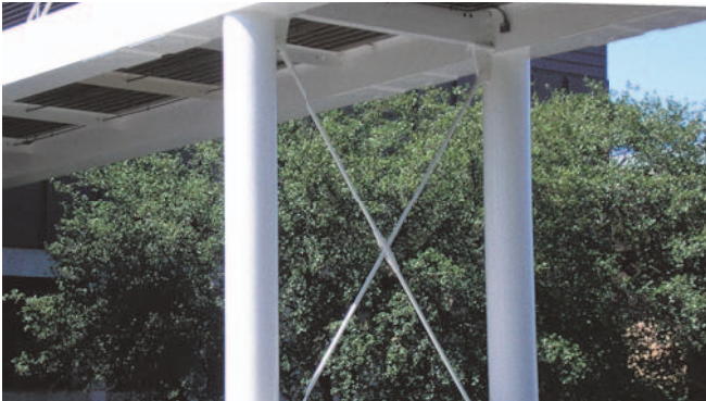
Cross-bracing with a cross coupler
