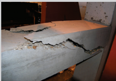
Post load test, showing ultimate shear failure mode; a continuous polystyrene strip was cast into the wall beneath the Ancon Eazistrip joint to simulate poor compaction of the concrete. The wall/slab connection remains essentially intact.
