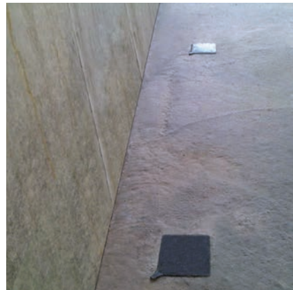
Void formers shown at Slab-to-Wall joint
