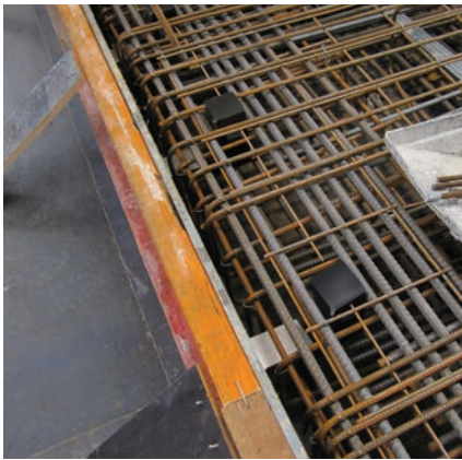
Reinforcement being located around ESDQ-L20 Sleeves
