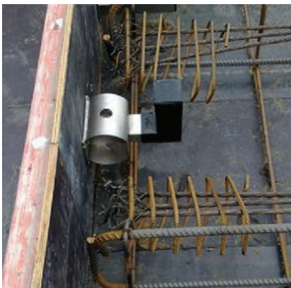
HLDQ-L30 Sleeve nailed to formwork
