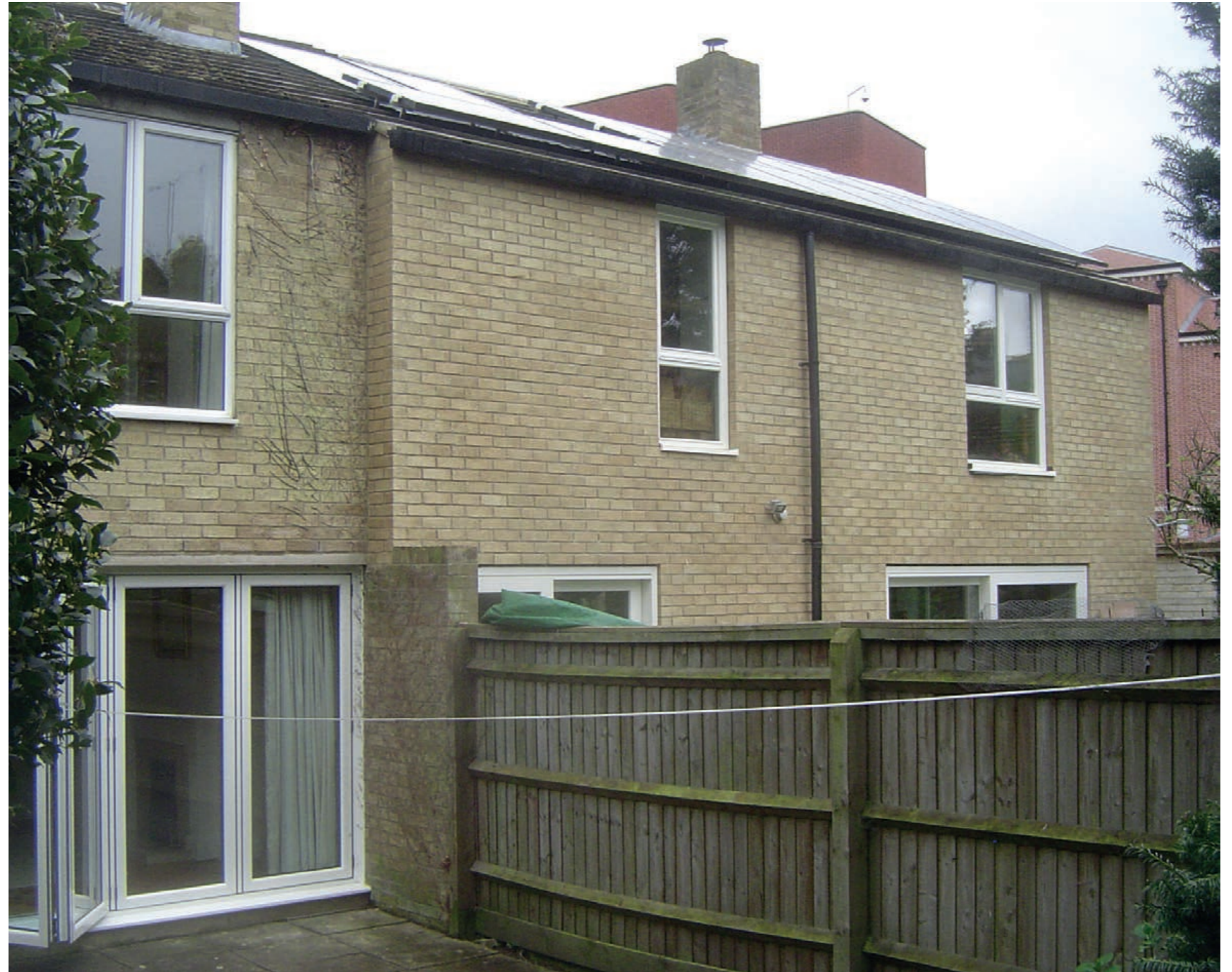
The new brick façade of 'The Oxford Greenhouse' is shown on the right, stepped 300mm off the façade of the neighbouring property.
