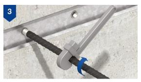
The Bartec Plus parallel-threaded continuation bars are inserted into the KSN Anchors and hand-tightened until fully locked using a wrench. Lap and fix the slab reinforcement and pour the concrete to complete the installation.
