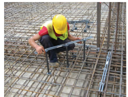
Radial Layout Installation
