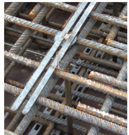
'Top down' installation. Rail is tied to the main reinforcement
