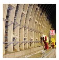
joined with a stainless steel retaining strip. In the event of a fire the integrity of the structure must be protected, and as temperatures could reach over 1000°C in the case of a fuel tanker incident, the tunnel lining is designed to keep the temperature within the tunnel below 300°C.
