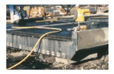
For a perfect fit with the adjacent slab, the endplates were supplied as match-drilled pairs. This guaranteed the precise positioning of 34 bolts at each shear connection. Our dedicated production team ensured all units were delivered to site over a 10 month period to suit the casting yard schedule.
