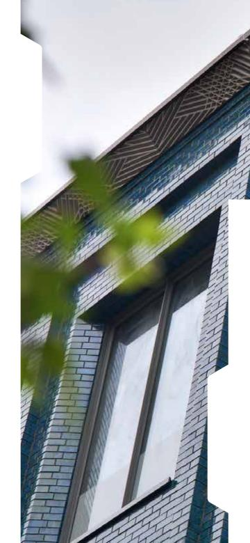
For ultimate durability, **NEXUS XI** has been engineered as a mechanical fix solution. This means that each individual brick on the suspended brickwork system is held in place using a combination of innovative fixing methods.
