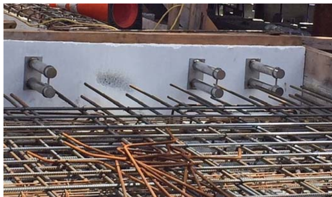
..... Modified DSD connectors showing clamped dowel bars.
