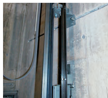
Elevator Guide Rail Connected using Cast-in Channels
