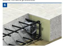
Now the reinforcement can be placed around the dowel, again paying attention to the reinforcement dimensions and the required concrete cover. The installation is completed by placing the concrete.
