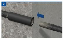
After casting of the concrete and when ready to extend, remove the plastic end cap from the coupler. Position the continuation bar in the sleeve and rotate the bar into the coupler.
