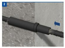
Position the continuation bar as near as possible to the coupler fitted to the cast-in bar.
