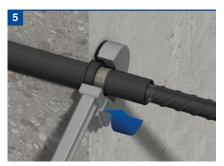
Run the locknut along the threaded barrel of the male component to abut the female section. Using the torque wrench, tighten the locknut to the specified torque. Tightening torques are shown in the table opposite.
